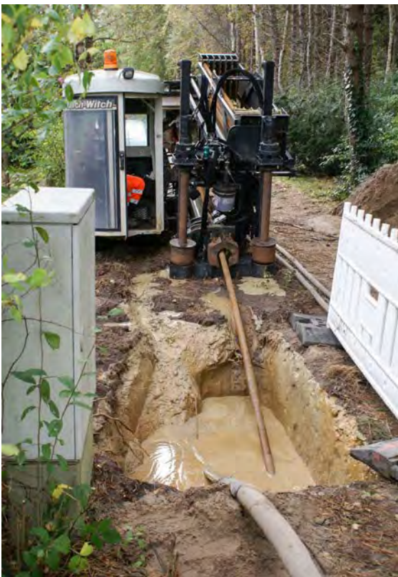
Fig. 07-13 RAUTHERMEX directional drilling
