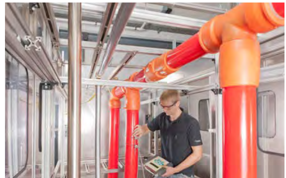
Fig. 06-21 Pipes and jointing technique are tested as a system
