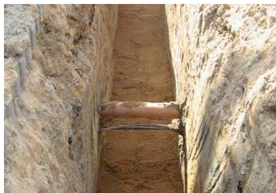
Fig. 07-2 Trench base with pipe support
