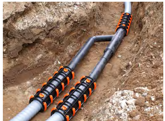
Fig. 04-34 Y-pipe installation in practice
