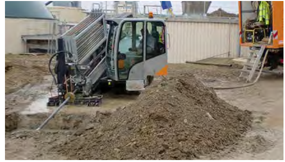
Fig. 07-10 Installation with horizontal directional drilling device
