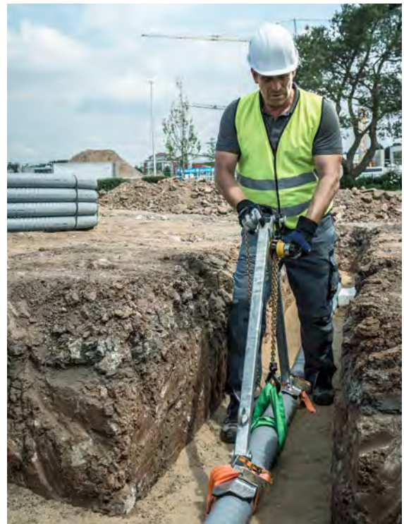
Fig. 07-38 STRAITA installation aid
