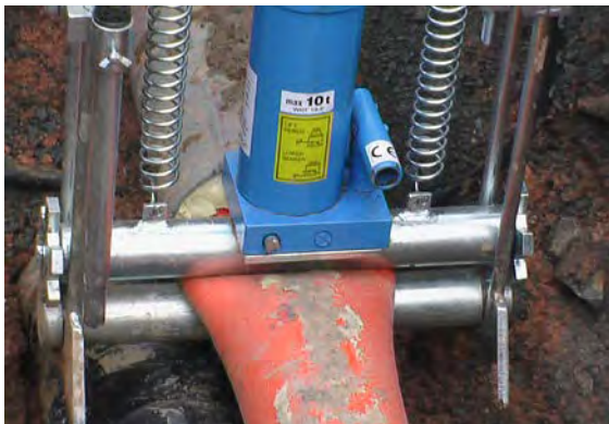
Fig. 07-31 Squeezing off UNO carrier pipes
