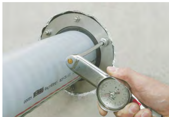
Fig. 05-12 Installation using a torque wrench
