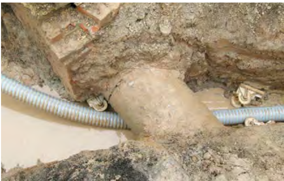
Fig. 07-24 Easy installation thanks to flexible pipe routing
