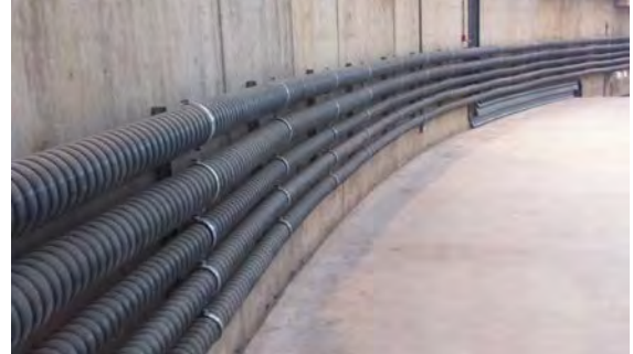
Fig. 07-28 Example of above ground / wall mounting
