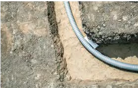
Fig. 07-23 Changes in direction without fittings
