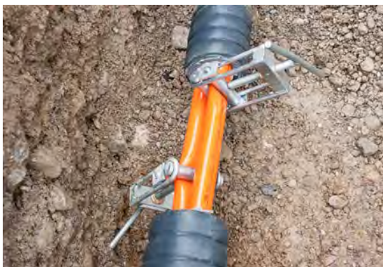
Fig. 07-32 Squeezing off DUO carrier pipes
