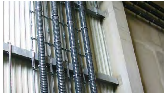
Fig. 07-29 Example of above ground/ wall mounting
