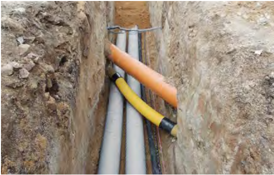
Fig. 07-22 Passing beneath crossing lines
