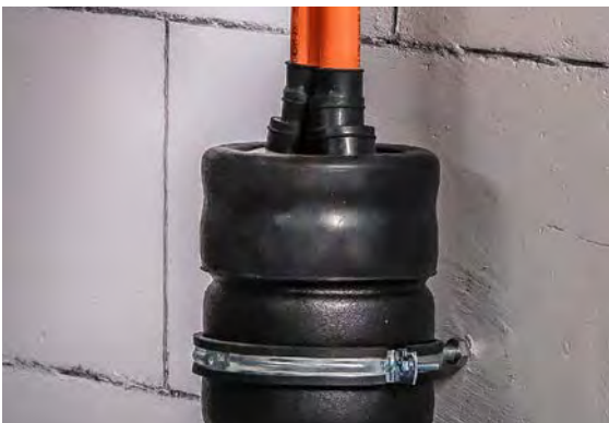
Fig. 05-23 Closing pipe with rubber end cap
