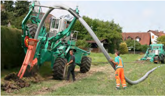
Fig. 07-8 Installation with mole ploughing machine
